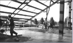
Radiant slab heat and air conditioning ductwork were installed. A pump truck with rigged scaffolding was used to deliver and evenly spread concrete over second story radiant floor piping.
