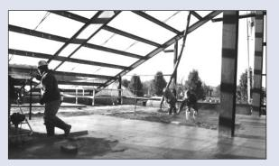
Radiant slab heat and air conditioning ductwork were installed. A pump truck with rigged scaffolding was used to deliver and evenly spread concrete over second story radiant floor piping.
