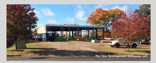
Work is also well underway on the building shell only construction of a medical office building for **Par One Development Company, LLC, in Stratford, CT.** The 10,240 SF building scope of work includes foundation, framing, parapet and cornice framing
